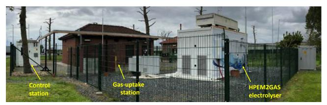
Fig.2 HPEM2GAS power-to-gas plant in Emden, Germany. On the right, the high performance 200 kW electrolyser from ITM Power based on Solvay Aquivion® membrane and CNR-ITAE electrocatalysts (HPEM2GAS project).
